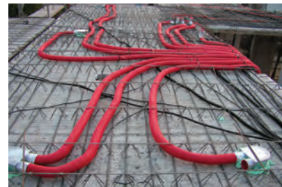
In the concrete screed
